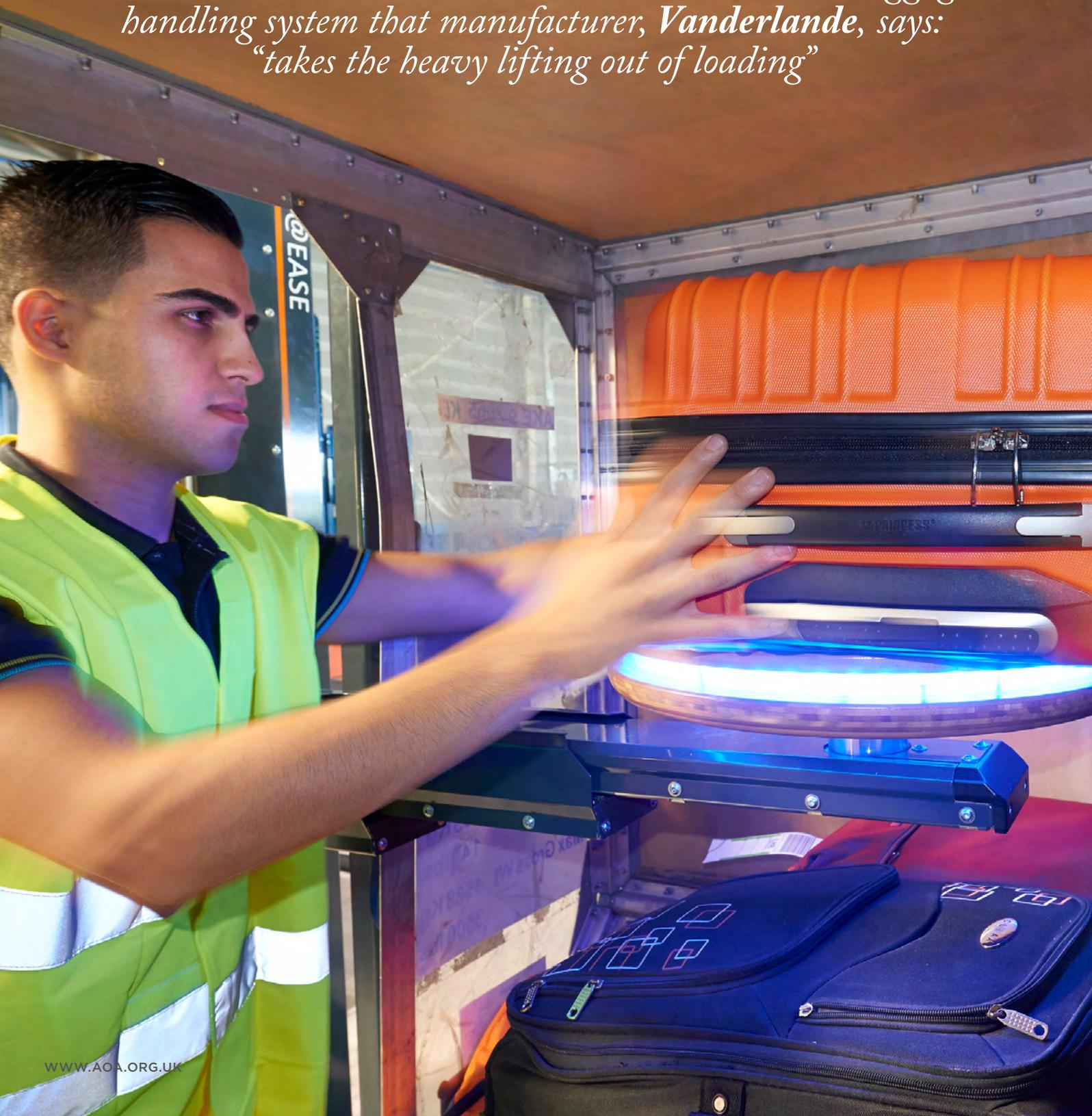
Following testing at Terminal 3 and Terminal 5, Vanderlande has supplied and installed 72 STACK@EASE units as part of the terminal's integrated baggage system. The new facility is the most advanced baggage system in Europe with a baggage handling capacity of up to 7,200 bags per hour. The system is designed to cut the time it takes to get bags ready for a flight to 90 minutes or less. Heathrow handles over 185,000 bags a day through a system comprising 30 miles of conveyors.
